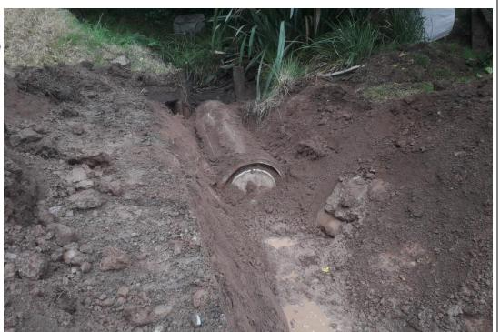
though, that one of these drums was firmly wedged in the culvert pipe; it was clogged to the hilt with mud and the source of flooding problem was found.
